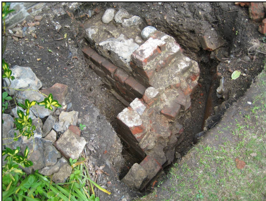
Fig. 8 - The excavated wall from the south A brick and a flint at the bottom are newer work built against a buttress of the main wall.
